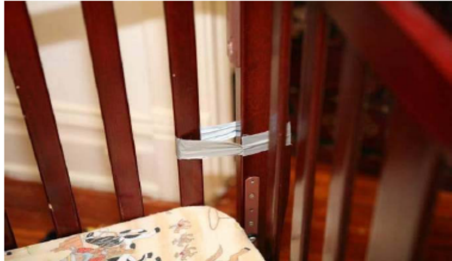
Homemade repairs to cribs like this one can be deadly.
