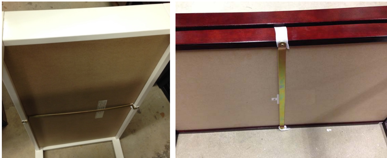
Figure 4: Examples of Secondary Support Straps Beneath Changing Surfaces
