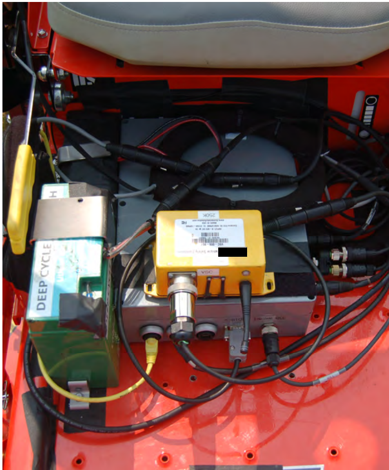
On-Vehicle Computer Box, 12V Battery, and Safety Circuit Box Mounted in Footwell of Vehicle
