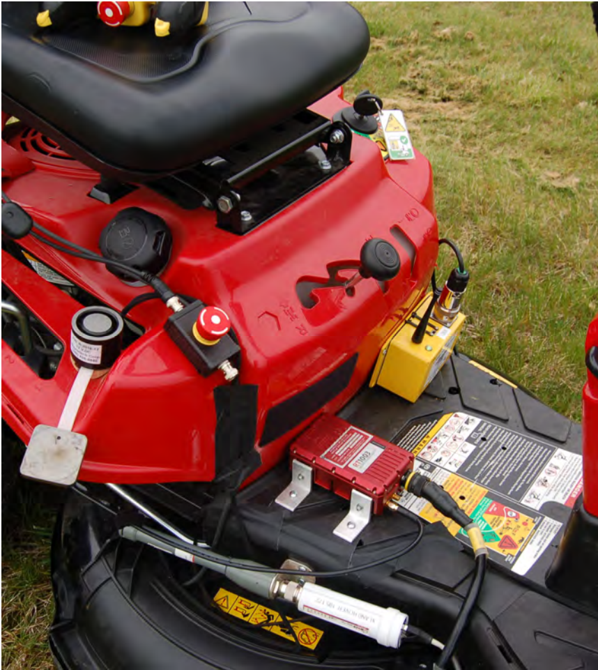
RT1003 GPS/IMU and Safety Circuit Box Mounted in Footwell of Vehicle
