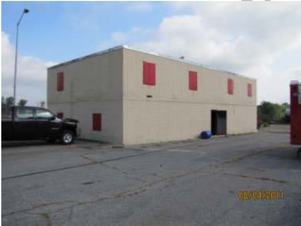
Figure 10. Exterior view of the burn prop building.
