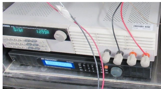
Power supply and load bank
