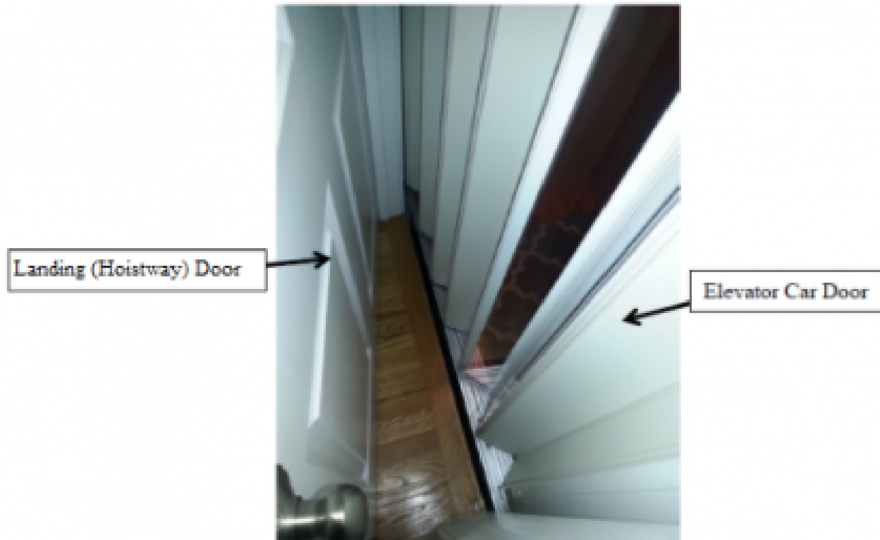
Typical Private Residence Elevator with Exterior Landing (Hoistway) Door and Interior Elevator Car (Accordion) Door
